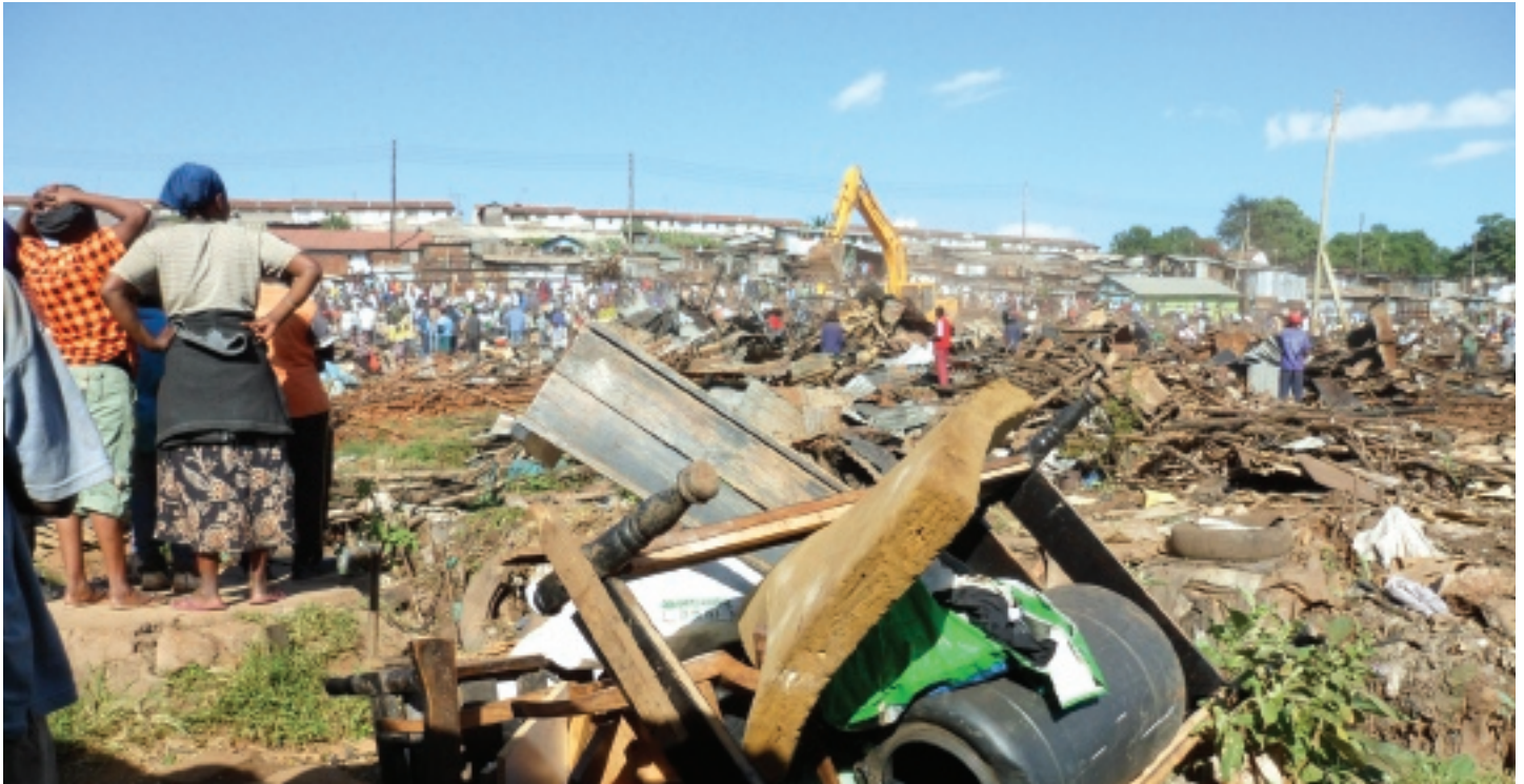
The destruction of demolition.
