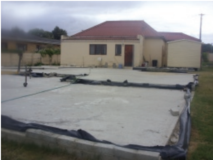
Building in Progress.
