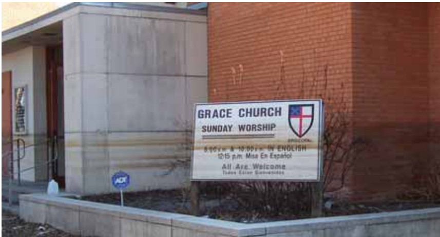
Flooded church: the water peak was about 4 feet higher than the line showing where it settled for over 2 weeks.
