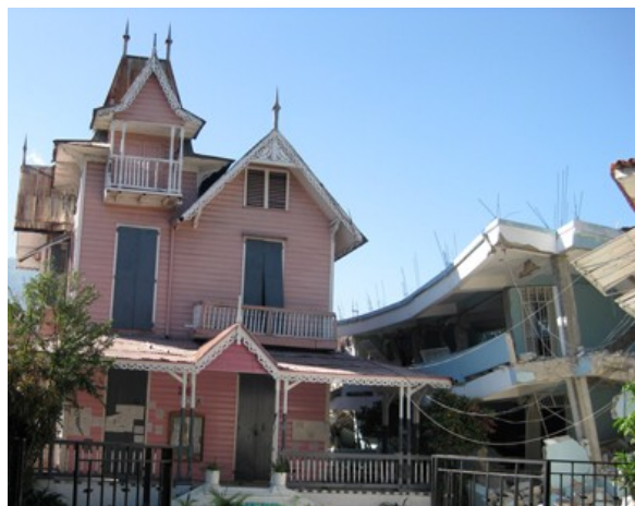
Only the old wooden administration building remains undamaged.
